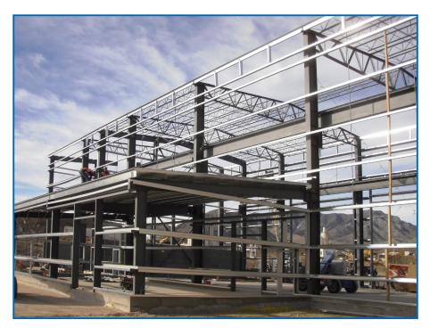
Three-dimensional model sharing prevented problems during the metal framing design and fabrication of a 12,600-square-foot Molycorp, Inc. truck maintenance facility in Mountain Pass, California.
