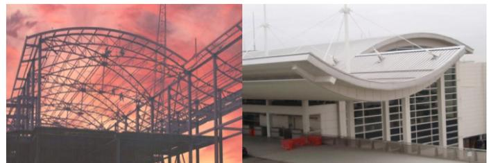
*Architect's vision of exposed truss was central to the interior design of the Detroit airport. The vision was cost-effectively achieved with engineered steel barrel joist systems. Finished airport roof, steel deck and support structure were the result of an upfront collaborative design process.*
