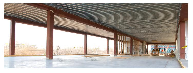
Structural building systems significantly affect your building's form, inside and out. For example, an architect envisioned this grand, 20-ft. wide hallway with an expansive feel. Load balancing was key to support the architect's vision. Taking an early design-assist engineering approach can ensure that support columns will not quash the architect's vision. A long-span composite floor system was used to meet the project requirements without obtrusive columns.
