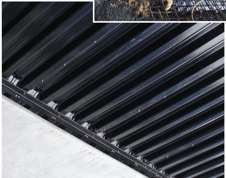
Rhino-Dek® polymer laminated stay-in-place forms protect bridges against corrosion, abrasion, and ultraviolet light.
