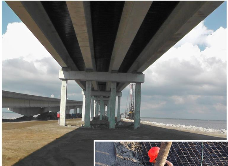
New Millennium's Bridge-Dek® and Rhino-Dek® stay-in-place steel form systems allow project owners to reduce costs by 20-25%, compared to wood forms.
