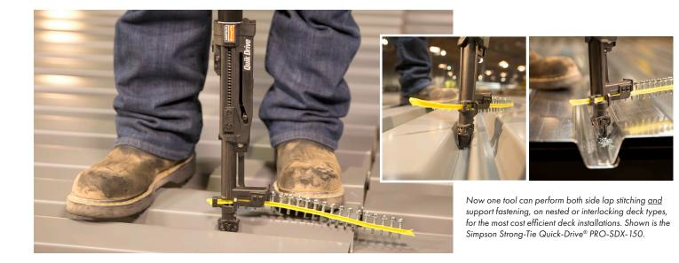
The installation trade has become increasingly aware of new steel deck installation tools that are automated and ergonomic, enabling faster, safer and lower-cost deck installation.
