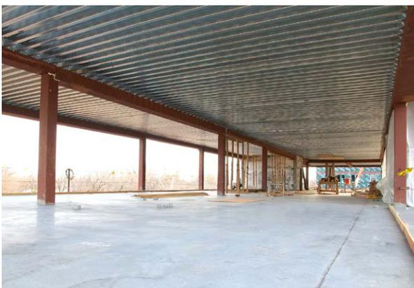
A long-span composite floor system was used in this 20-ft wide hallway to meet the architect’s vision without obtrusive columns.
