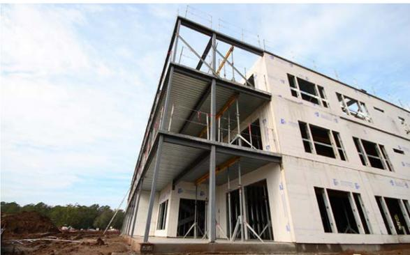
*The Versa-Dek® system permits an open-floor plan design with the required strength to withstand the elements.*
