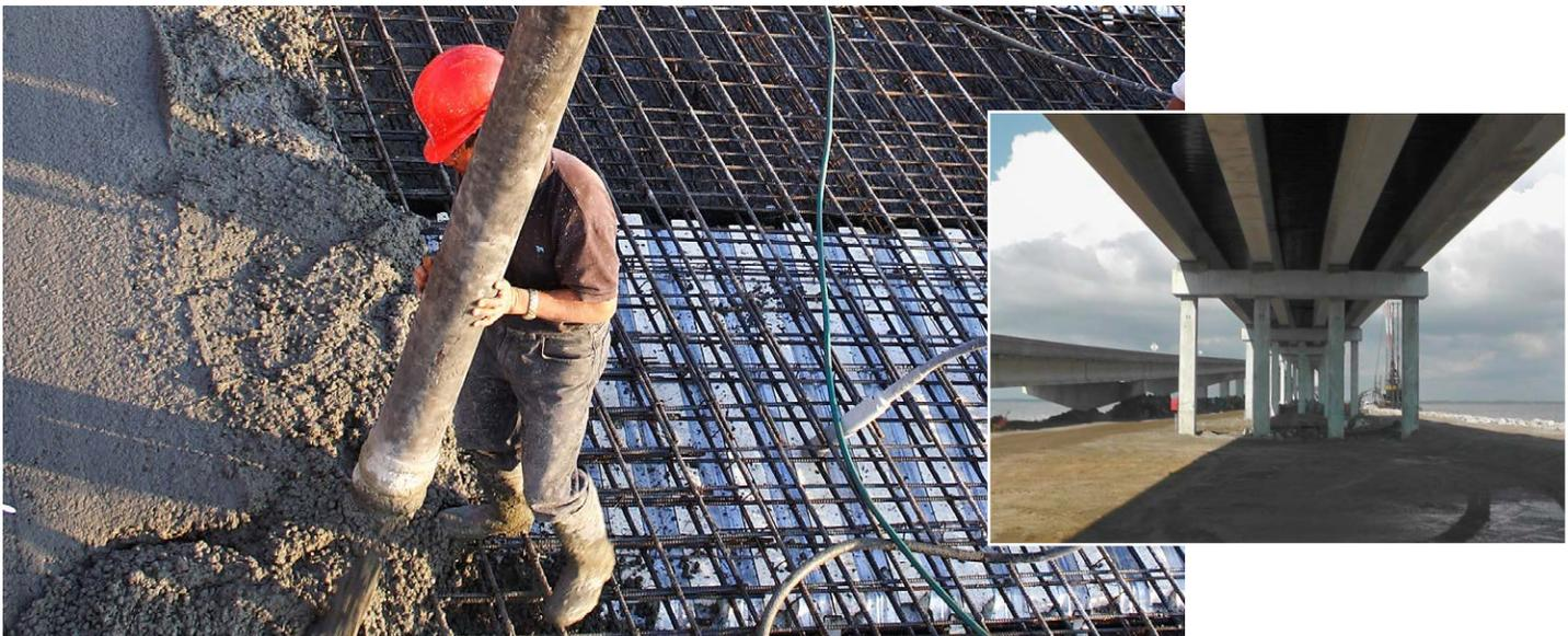
New Millennium’s Bridge-Dek® and Rhino-Dek® stay-in-place steel form systems allow project owners to reduce costs by 20-25%, compared to wood forms.
