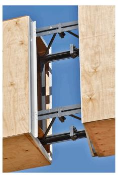
The bridging between the barrel joist trusses connect them all to provide support in more than one direction on the Ford dealership brand wall application.
