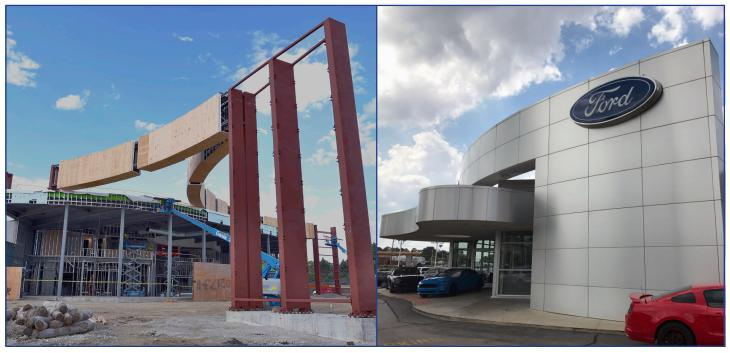
Barrel joists cladded in plywood and connected by custom trusses span the roof of a car dealership under construction (left) and will resemble this previously completed design (right).
