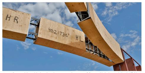
New Millennium delivered the barrel joist box trusses to the customer fully assembled, along with detailed field drawings to aid in proper installation to speed erection and ensure correct and safe on-site construction.
