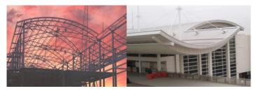
Architect's vision of exposed truss was central to the interior design of the Detroit airport. The vision was cost-effectively achieved with engineered steel barrel joist systems. Finished airport roof, steel deck and support structure were the result of an upfront collaborative design process.
