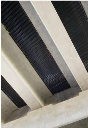
All deck and accessories are fabricated from steel conforming to ASTM Specification A-653 Grade 50 having a minimum coating class of G165 according to ASTM Specification A-924. The steel unit working stress will not exceed 0.725 of the specific minimum yield strength or a maximum of 36,000 psi.
