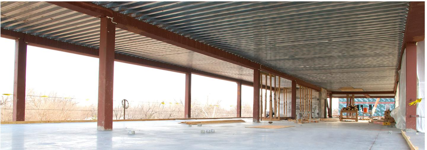
Structural building systems significantly affect your building's form, inside and out. For example, an architect envisioned this grand, 20-ft. wide hallway with an expansive feel. Load balancing was key to support the architect's vision. Taking an early design-assist engineering approach can ensure that support columns will not quash the architect's vision. A long-span composite floor system was used to meet the project requirements without obtrusive columns.
