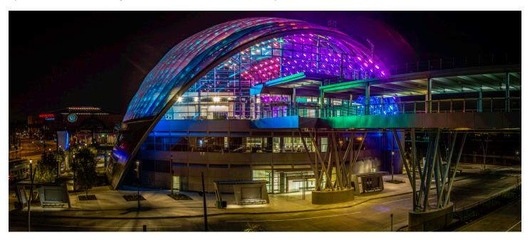
The Anaheim Regional Transportation Intermodal Connector (ARTIC) lights the way to more efficient urban transportation. Multi-colored LEDs inside an EFTE membrane creates a welcoming beacon for travelers. Here you will see another enlightened design idea: Exposed long span steel decking.
