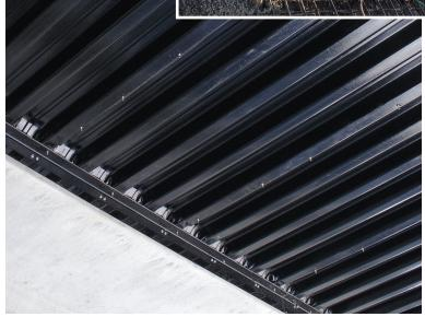
Rhino-Dek® polymer laminated stay-in-place forms protect bridges against corrosion, abrasion, and ultraviolet light.
