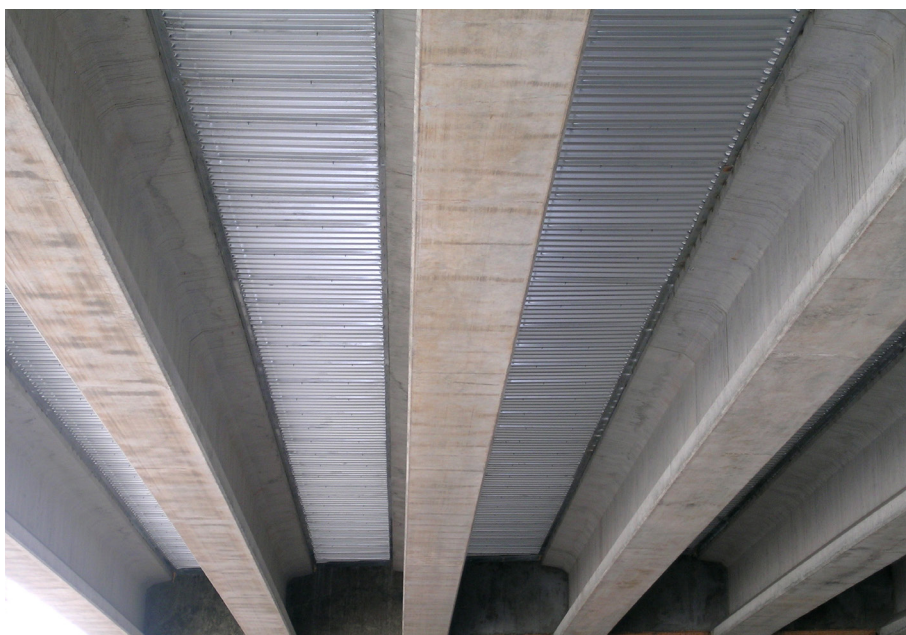
The four standard profiles of New Millennium's Bridge-Dek® and Rhino-Dek® solutions.
