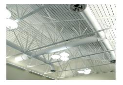
The raw, industrial look of an overhead painted and exposed steel joist/deck system, with pipes and HVAC ductwork woven through the joist diagonal web members, can often support both the roof of a building and the brand image of the occupying business.
