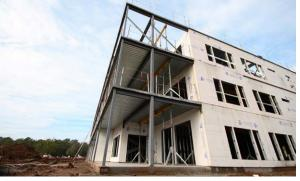
The Versa-Dek<sup>®</sup> system permits an open-floor plan design with the required strength to withstand the elements.
