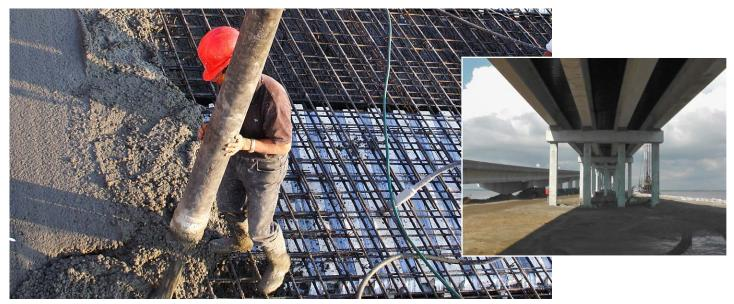
New Millennium's Bridge-Dek<sup>®</sup> and Rhino-Dek<sup>®</sup> stay-in-place steel form systems allow project owners to reduce costs by 20-25%, compared to wood forms.
