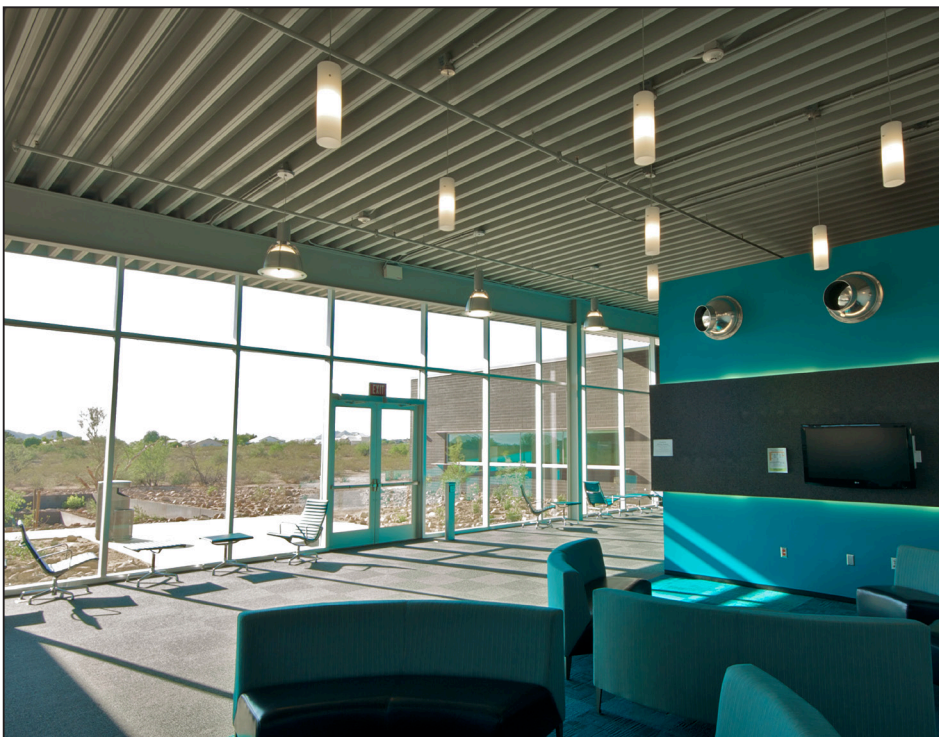
While transitioning areas of study to inspiring desert views, the steel roof decking addresses the unique acoustical and environmental challenges posed by the desert environment. The decking was engineered and manufactured by New Millennium. The general contractor on the project was CORE Construction. The architect was RNL Design.
