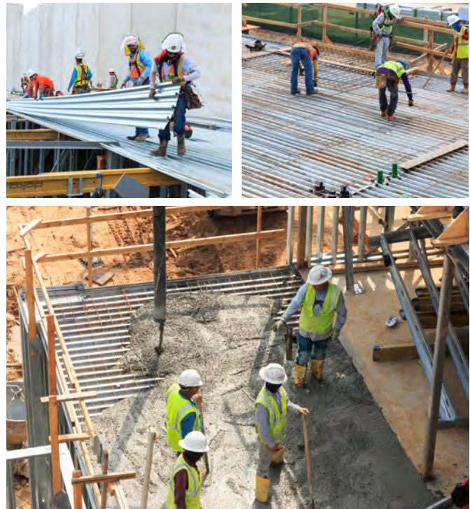
Deck installation, slab reinforcement placement and concrete casting incorporate traditional equipment and methods.
