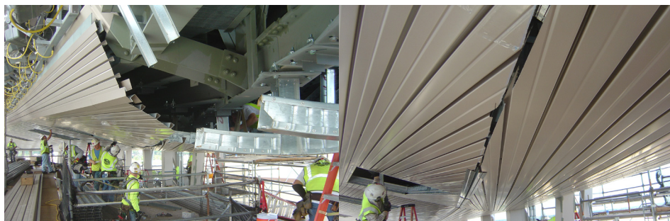
The compound curvature of the stadium's canopy was easily followed using flexible Versa-Dek® dovetail steel decking. Fasteners are concealed inside the decking's dovetail profile.
