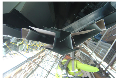
Custom-designed trim pieces feature slotted expansion joints to allow the sections to shift with Minnesota's extreme temperature variances.
