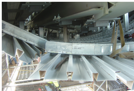
The compound curvature of the stadium's canopy was easily followed using flexible Versa-Dek® dovetail steel decking. Fasteners are concealed inside the decking's dovetail profile.
