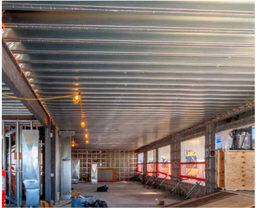
Another example of Deep-Dek® Composite integrating into existing framing structure is this 11-story Brooklyn multi-family residential building combining structural steel frame and CFS bearing walls.
