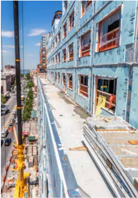
Another example of Deep-Dek® Composite integrating into existing framing structure is this 11-story Brooklyn multi-family residential building combining structural steel frame and CFS bearing walls.
