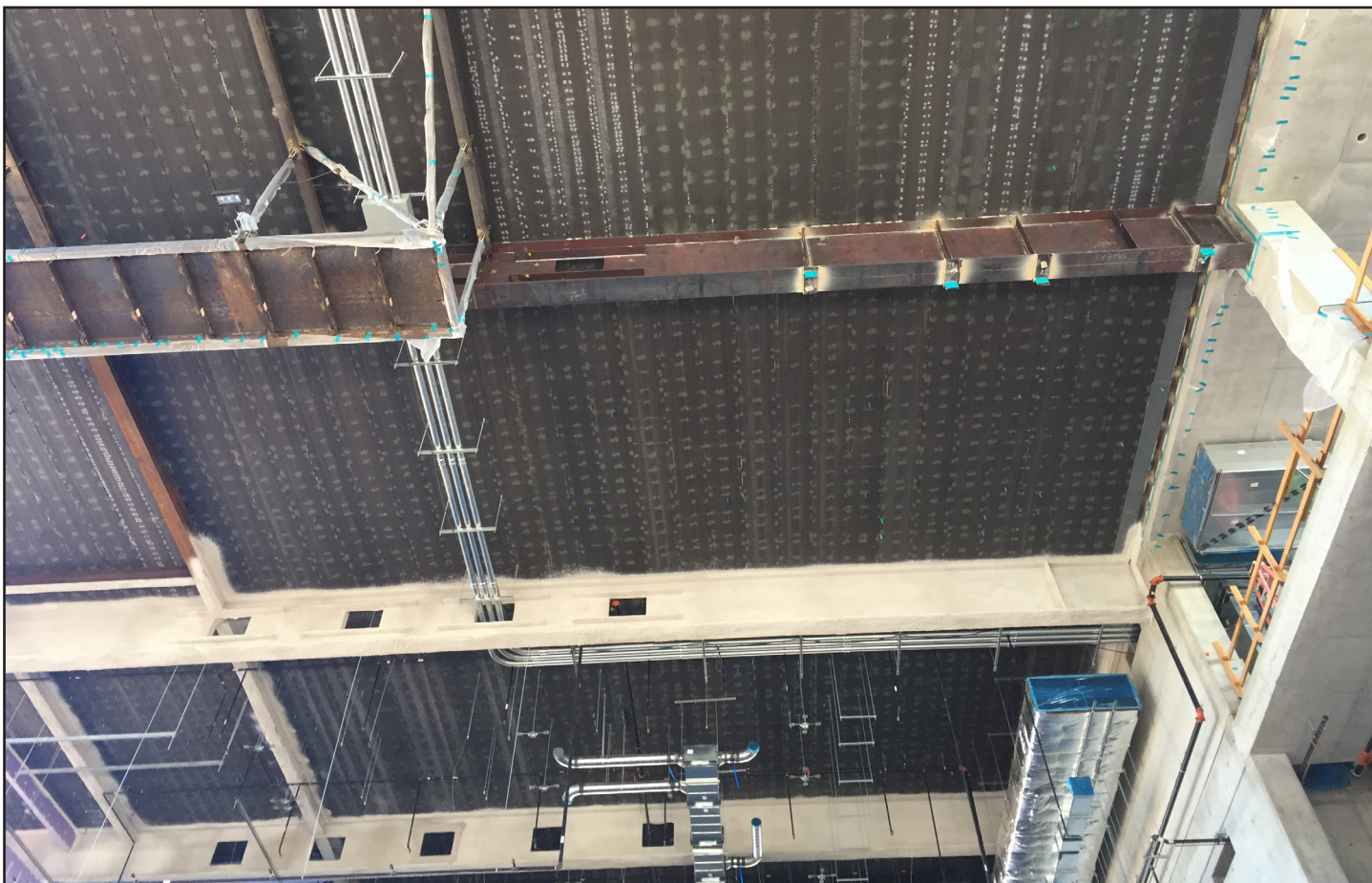
MEP pass-throughs, embedded electrical boxes, and slab penetrations were carefully designed and coordinated.
