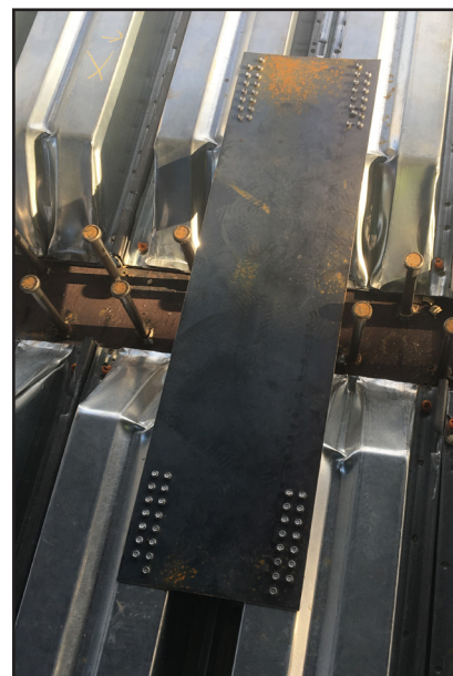
Shoring was eliminated by the installation of continuity plates to bridge the deck ends on both sides of the girder beams.
