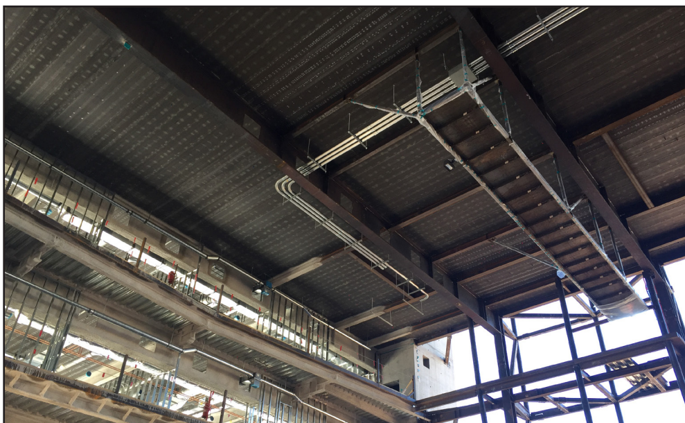
The massive, open-learning space in the center of this 220,000 square foot learning facility was framed using long-span composite floors to create thin slabs that are set on 80-foot-long plate girders. Shoring during floor construction was not an option, so a creative solution was required.
