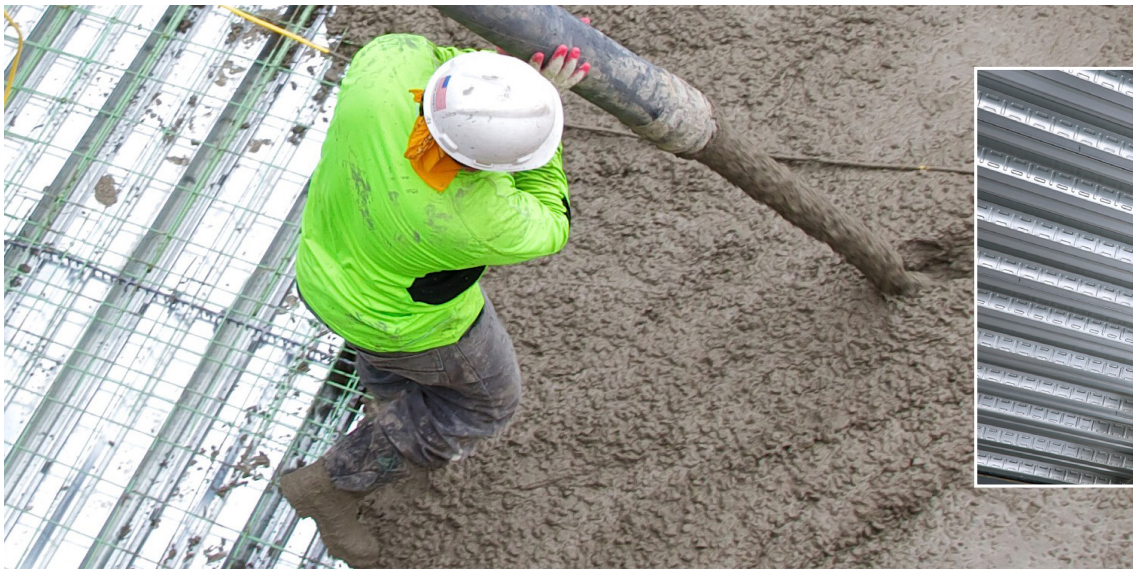
Composite steel deck is made by roll-forming structural grade steel into a repeating pattern of parallel ribs. The concrete bonds to the ribs, providing structural strength and rigidity.
