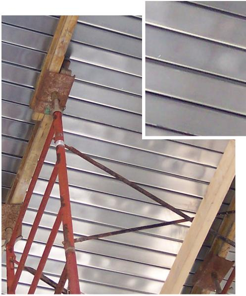
As seen here, oil-canning, or stress wrinkling, is an unsightly problem associated with several different causes but avoidable with the use of longitudinal stiffeners
