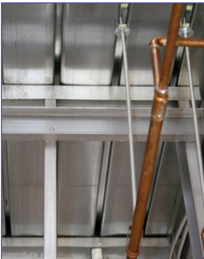
This Versa-Dek® Composite floor system installed in a multi-story residential project features the Versa-Wedge® system to hang MEP conduits.
