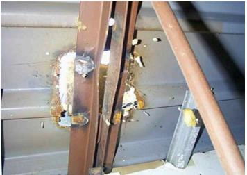
For reasons demonstrated by the photos above, the attachment of fall arrest anchorage or screen posts to the top chord of a joist is not recommended. Lateral bending forces in conjunction with poor field welding can result in post tear-off, as was the situation shown at left. The photo on the right shows the underside view of the joist top chord after post connection failure.
