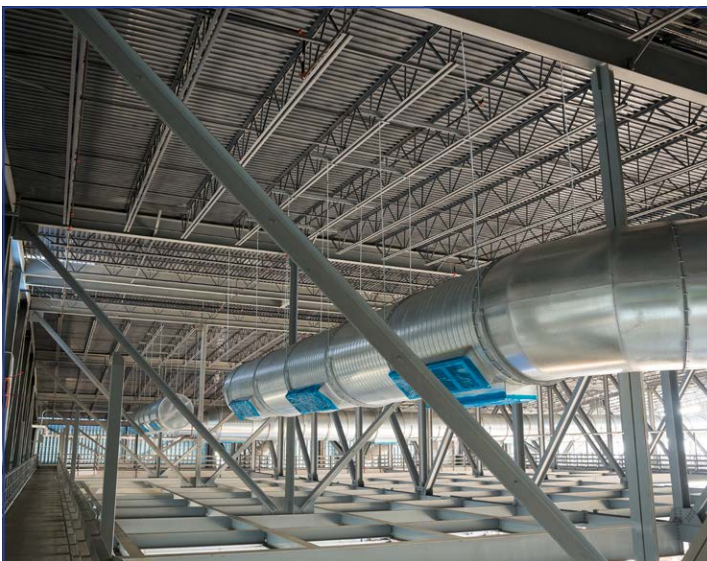
Steel Joists, Joist Girders, and trusses provide optimum integration of MEP systems.
